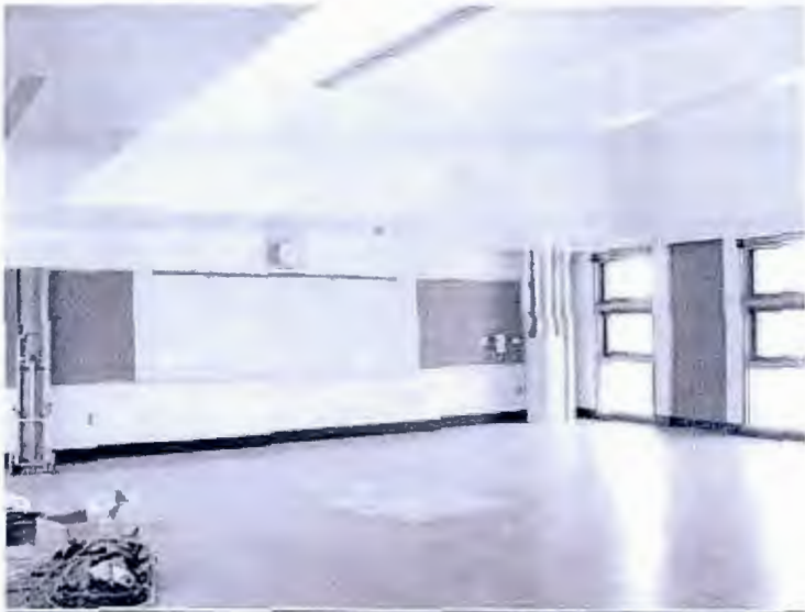
Typical 2nd story classroom @ Highland (Construction Photos)
