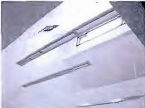
Roof monitors, shades open
