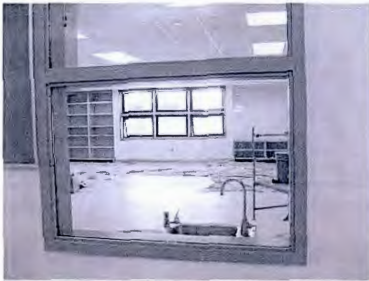
Interior corridor window shares daylight with classroom @ Highland Elementary
