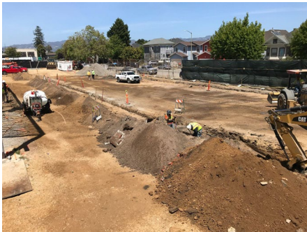
Image 1: Excavating for telecommunications trench in parking lot.
