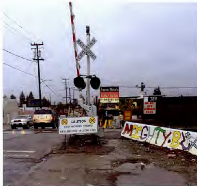
Figure 12: 105th Avenue Crossing, Looking North on East Side of Street
