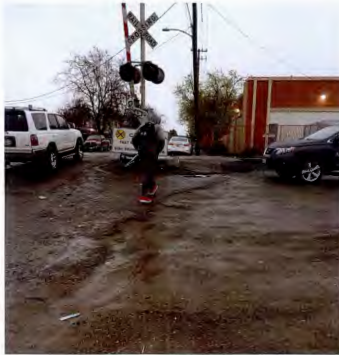
Figure 11: 105th Avenue Crossing, Looking South on West Side of Street
