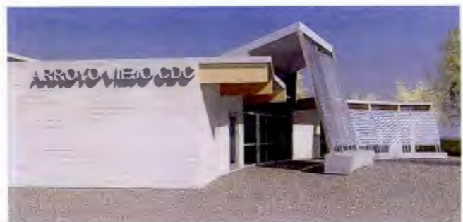
Arroyo Viejo CDC Renovation
