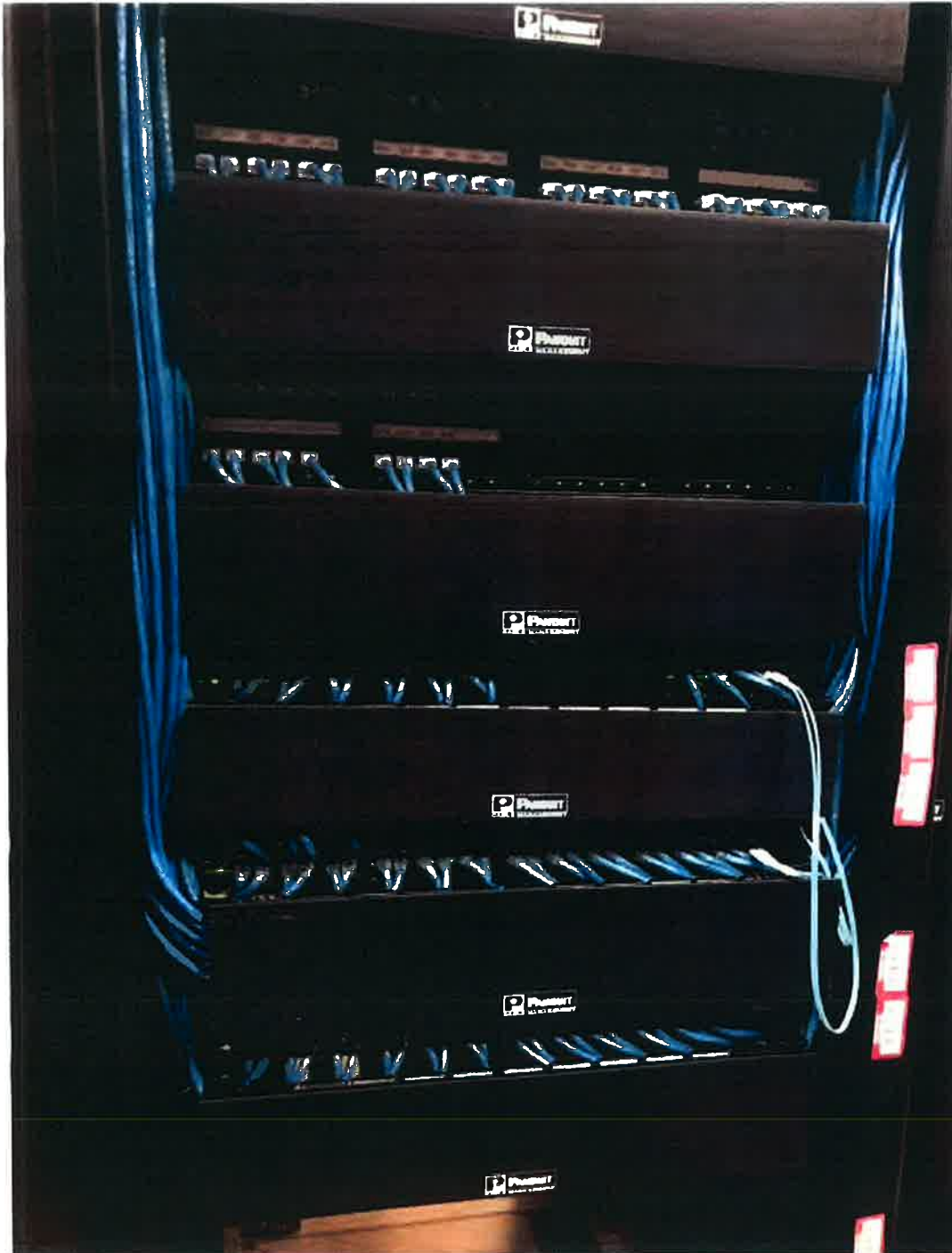
Example 4: Panels labeled, cables are neat, equipment is spaced properly
