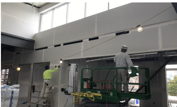
Image 02: Subcontractors applying drywall tape
