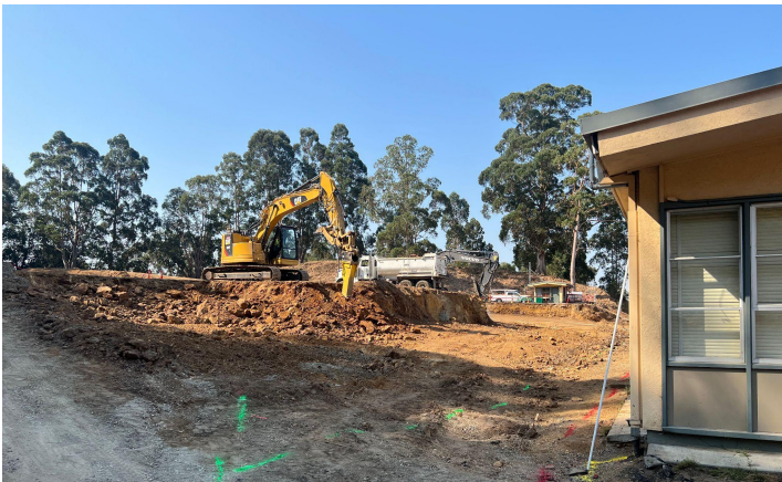
Image 01: Site work preparations for outdoor area
