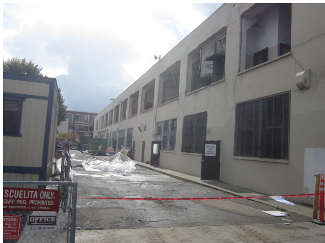
Harper Building (To be demolished)
