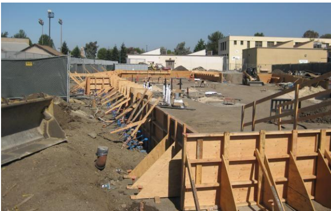
Concrete Form Work
