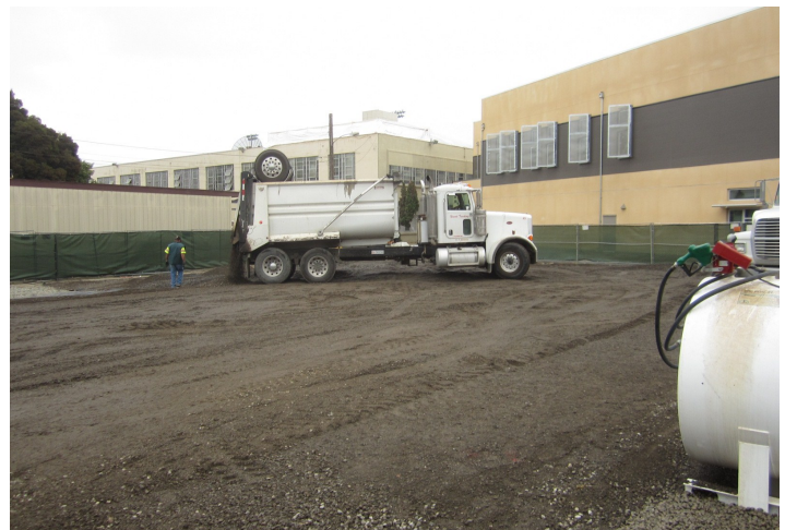
Site Preparation for Phase 2
