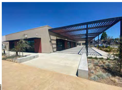
(Administration/Classrooms trellis shown above.)
