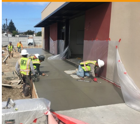
Pathway/ sidewalk at Training Classroom
