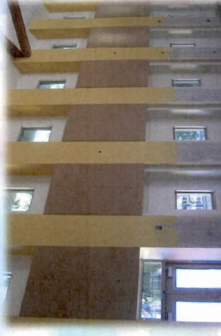
Progress Photos – Multi Purpose Bldg.
