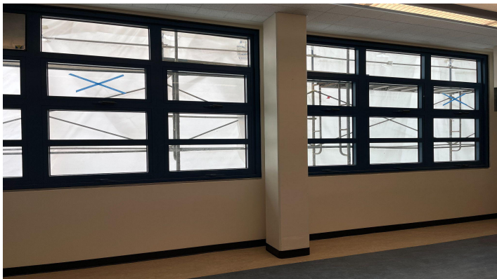
Classroom interior with window replacement
