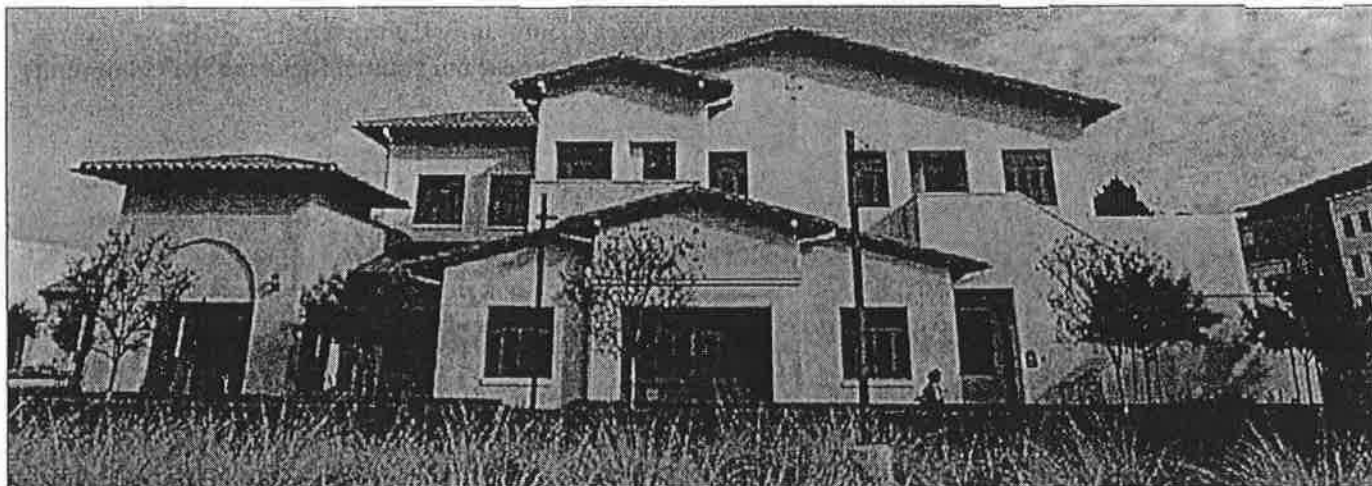
Building V at the Liberal Arts Campus is the new home for the Culinary Arts Department and the Math Department.
