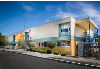
Laurel Elementary School
