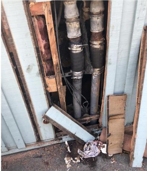
Leaky and rusted boiler pipes at MLK
