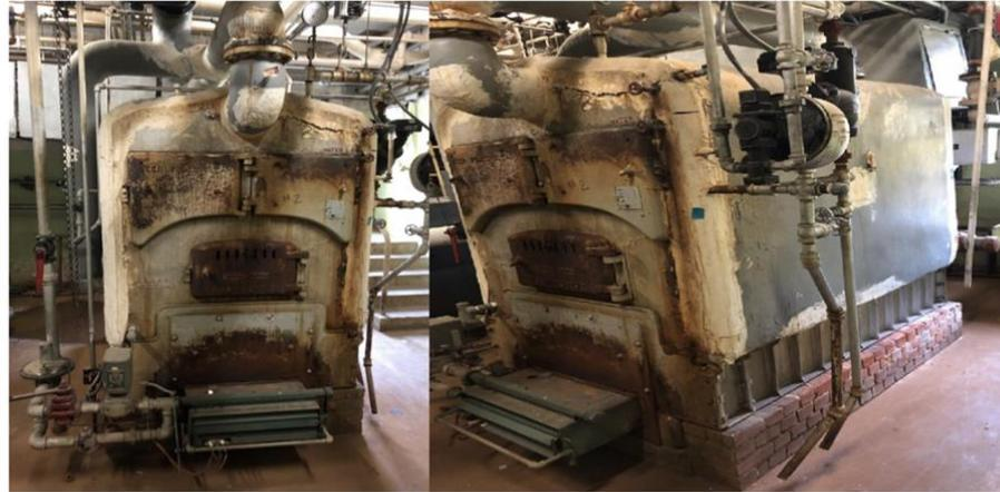
Fruitvale boiler from 1946. It is rusted and only one works
