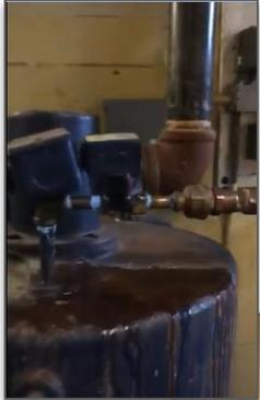
Multiple areas of boiler leaking when providing heat to classrooms
