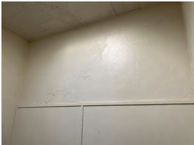
Photo 23: Academic unit stairwell water damage in plaster
